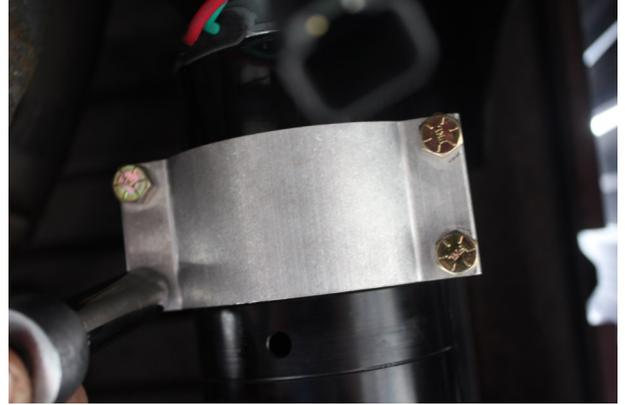
**VERY IMPORTANT: REMEMBERING THE POSITION OF THE "T" PORT, THERE IS A SMALL WEEP HOLE IN THE BASE DIRECTLY NEXT TO THE ELECTRIC MOTOR, THIS HOLE MUST AIM DIRECTLY TO THE GROUND!! IMPROPER INSTALLATION OF THE PUMP CAN CAUSE PREMATURE WEAR AND VOID MANUFACTURES WARRANTY.**
